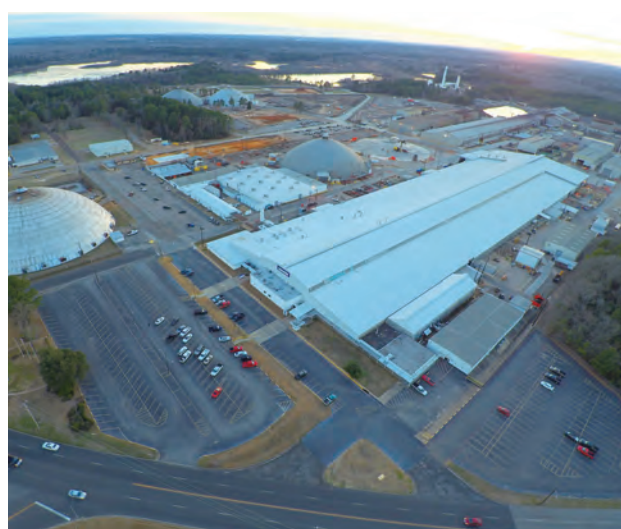
KMC Longview, TX Facility
