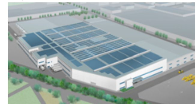
New Awazu Assembly Plant
