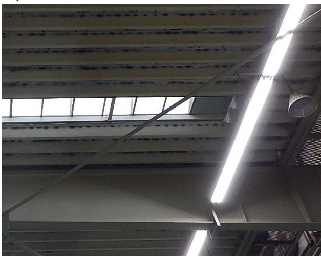
Ceiling lighting and modulated LEDs
