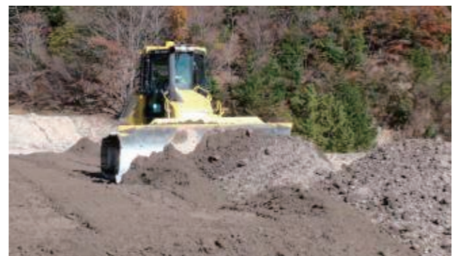
Construction under fully-automatic control (ICT construction equipment)
