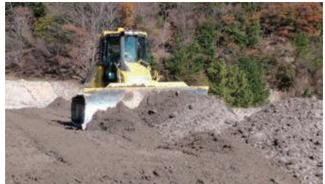
Construction under fully-automatic control (ICT construction equipment)
