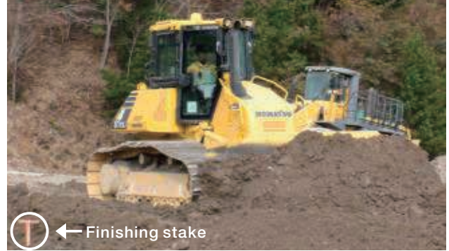
Construction in a manual operation in which finishing stakes are checked visually (previous procedure)
