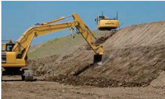
Construction under semiautomatic control [Slope trimming] (ICT construction equipment)
