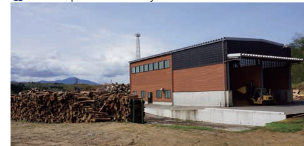
Woodchips Production Building and Lumber for Woodchips
