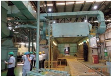
Environmental Inspection at BKC
