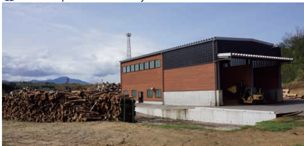
Woodchips Production Building and Lumber for Woodchips
