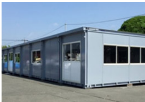
Temporary house put up as the temporary town office building
