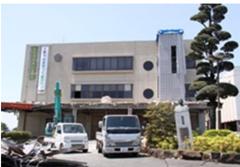
Mashiki town office building damaged by the earthquake
