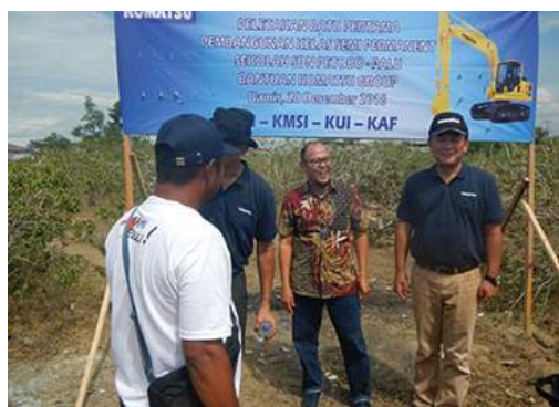
Construction site of an elementary school in Sulawesi
