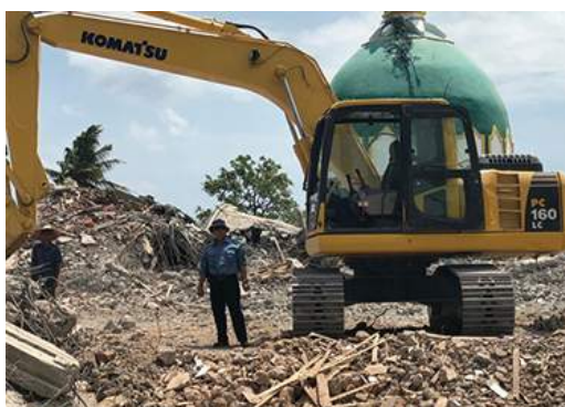
Hydraulic excavator in the Lombok Earthquake-stricken area
