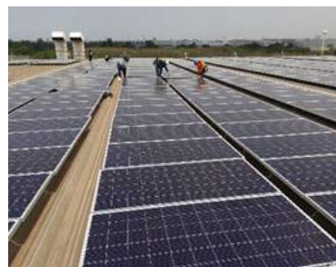
FY2018: solar roof under construction
