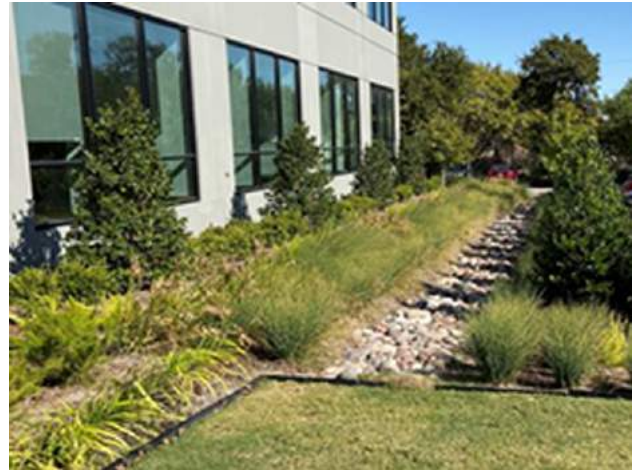
Hensley's Dallas facility : Bioswale
