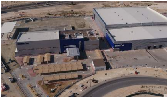
The Dubai Training & Demonstration Center
