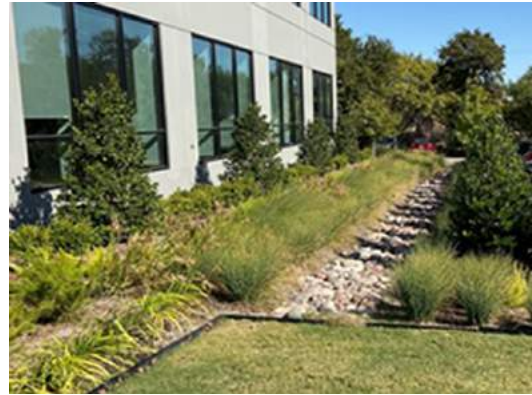
Hensley's Dallas facility : Bioswale
