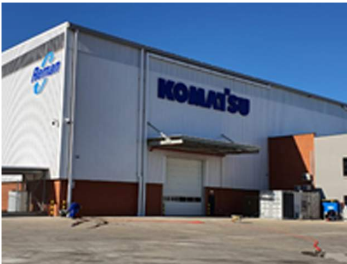
Komatsu Africa Holdings' new Reman building
