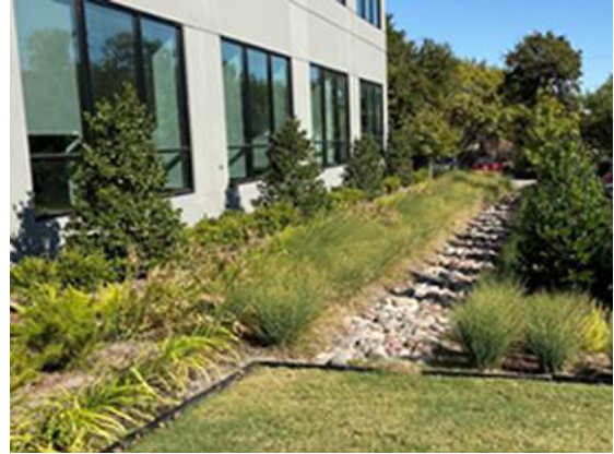
Hensley's Dallas facility : Bioswale
