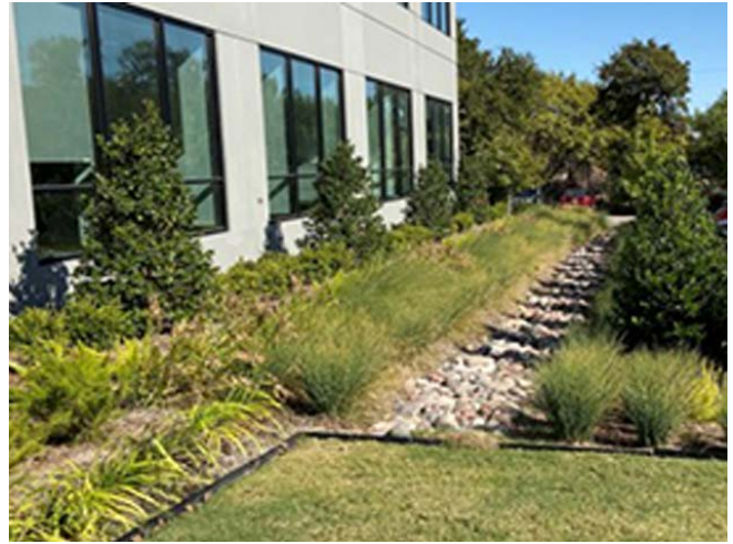
Hensley's Dallas facility : Bioswale
