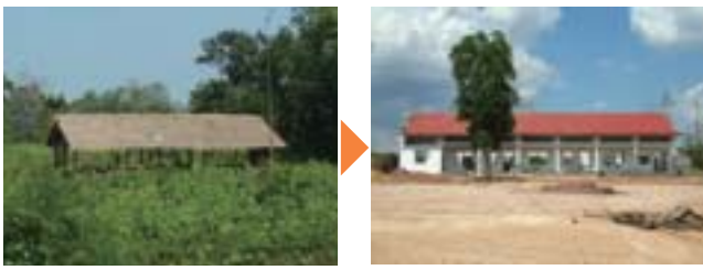
(Left) An elementary school surrounded by mined fields. After demining, a new school building and school grounds were constructed. (Right) The new school building is made of concrete and its foundation is raised off the ground, enabling the children to study without worry even in the rainy season.
