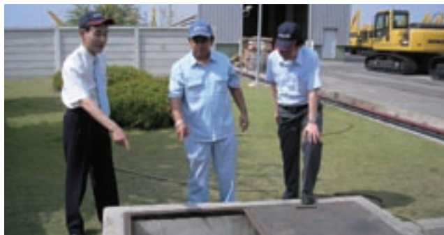
Guidance in maintenance of a separation tank (Bangkok Komatsu Co., Ltd.)
