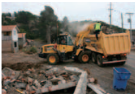
Loading rubble into a dump truck
