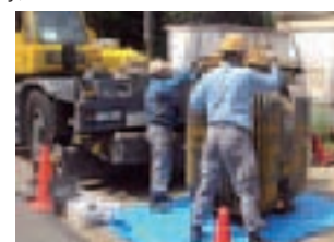
Transformers being removed from the Osaka Plant for disposal
