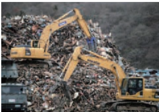
Hydraulic excavators at work in stricken area
