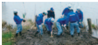
Pond excavation (47 newly hired employees participated)
