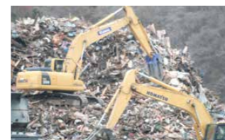
•• Hydraulic excavator in operation in Onagawa, Miyagi Prefecture, where removal of debris was a pressing need
