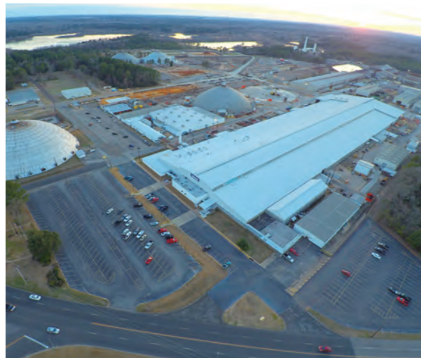
KMC Longview, TX Facility
